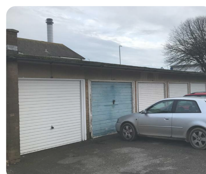
Coates Court garage area - Access from Butts Road
